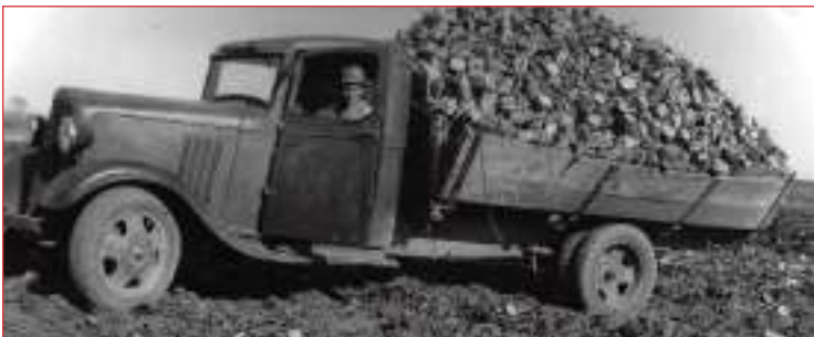
Beet truck boxes were widened to get more sugar beets on a load. Note the chain dangling from the front side of the box. There were generally more chains to hold the box in the extended position. 1934 Newell Museum
