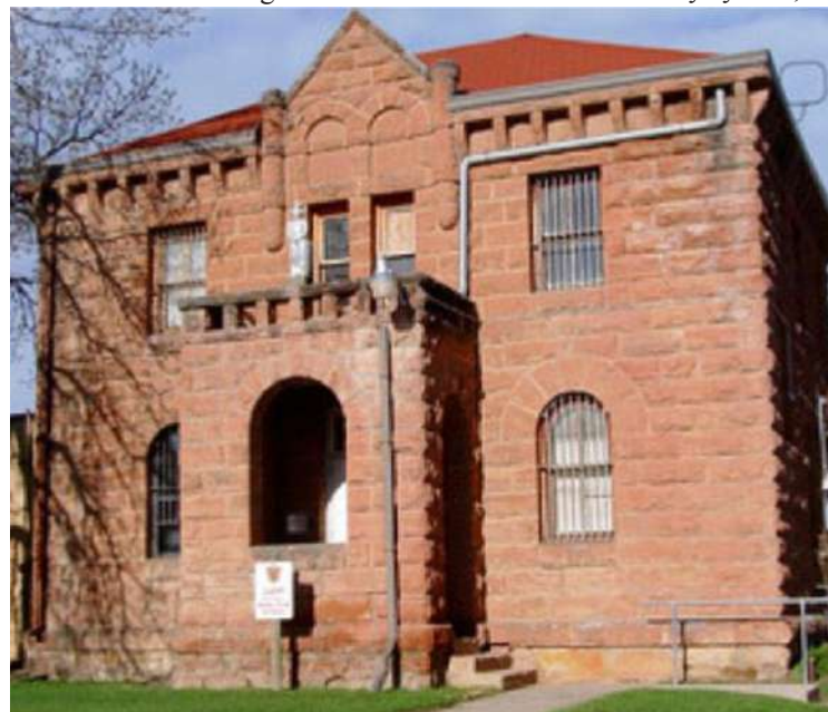
Butte County former jail, built ca 1897 listed in the Register of Historic Places. The availability of natural stone in western South Dakota contributed to the masonry tradition that developed in this part of the state. Sandstone was quarried at areas of natural outcropping in Butte county and was used for construction of massive public building.
